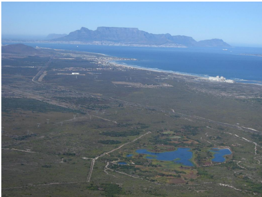
Infiltration Basin 7 at Atlantis Water Resource Management Scheme
