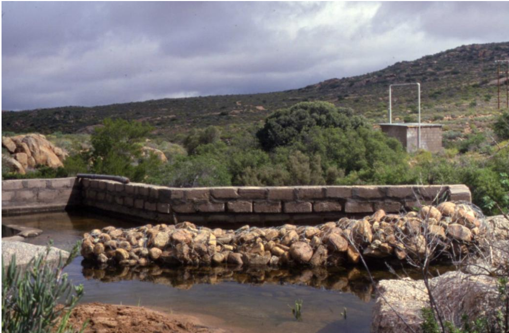
In-stream filter upstream of Kharkams' artificial recharge borehole
